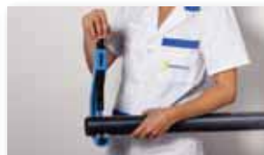
Cut the pipe with the pipe cutter.
