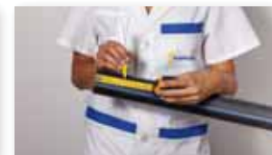
Mark the area to be scraped.
