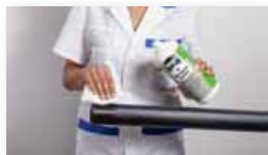
Use the proper scrapers. Clean the surfaces with a suitable detergent.
